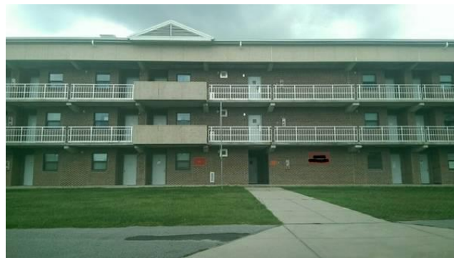
A 20 JUL ad for a room in the Marine Corps barracks at Camp Lejeune, N.C., touts laundry in building, "motivation specialists" and early wake-up calls.
