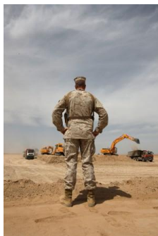
A U.S. Marine watches as a construction crew works on a new base at Camp Letherneck in Afghanistan.
