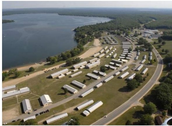
Maintenance facility at Camp Grayling, in Grayling, Mich.
